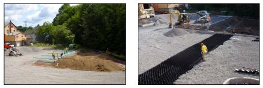
Figure 3.8 Installation of porous pavement at the WAP Office in Tannersville
