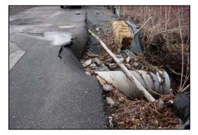
Stormwater runoff from Garfield Road east of the intersection with Point Breeze Drive and runoff from Prince and Lookout Mountain Drive currently discharge directly to the Schoharie Creek via a culvert underneath Route 23A. Within this drainage area there are five swales and five culverts that represent potential stormwater runoff sediment sources.
