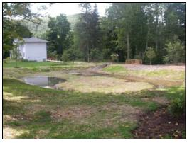
Stormwater wetland in center of photo, permeable parking area to the left and kiosk behind the wetland.
