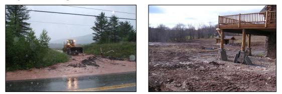
**Figure 7.2 Examples of Construction Practices without Stormwater Controls**
