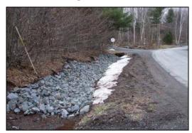
Erosion zone on Pine Lane from undersized culvert caused this ditch to be armored with stone
