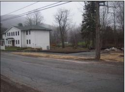
Partially completed permeable parking area. Stone subbase, topped by geoweb filled with soil and stone.
