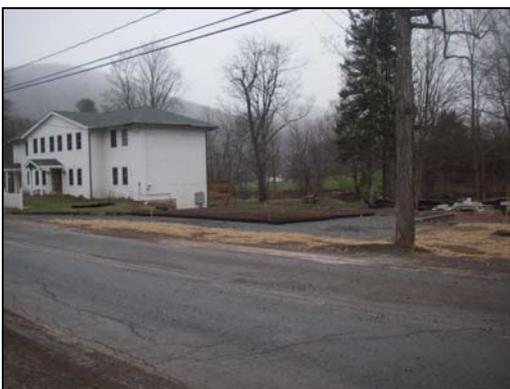
*Partially completed permeable parking area. Stone subbase, topped by geoweb filled with soil and stone.*
