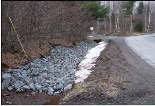
*Erosion zone on Pine Lane from undersized culvert caused this ditch to be armored with stone*
